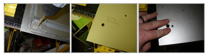
• Using the flag as a guide to where to drill the holes. Mark a spot for a hole for the flag to go through in the door of the case. Then drill holes accordingly.
