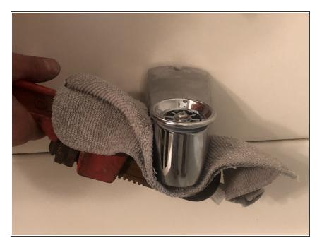
Once too tight to continue twisting, place a rag around the spout and continue to twist with the pipe wrench clockwise (to the right) until fitted against the wall.
