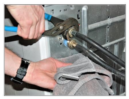
Disconnect the supply hoses using channel lock pliers. Use the towel to catch any water that may spill out.
