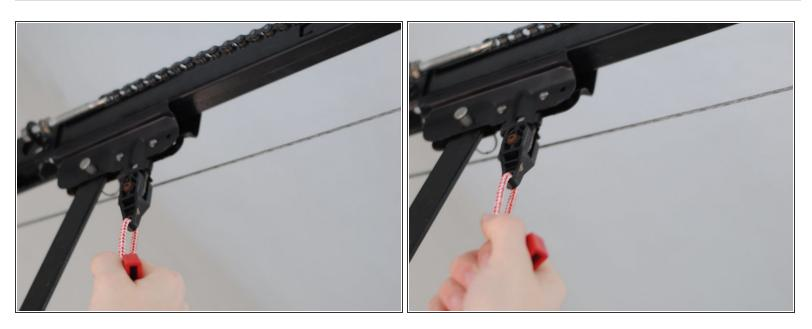
There is a handle located at the top of the door for manually releasing the door from the chain rail.
