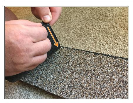
Remove the adhesion strip off of the new shingle.
