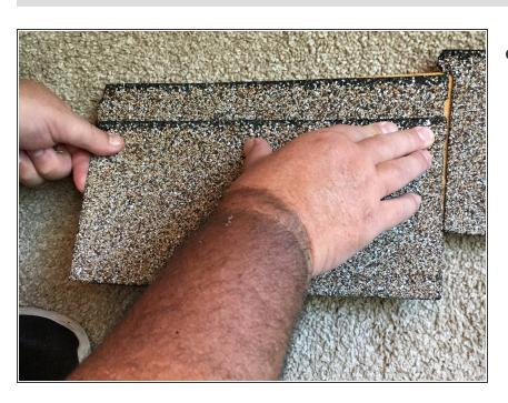
Press down the edges to lock the shingle in place.
