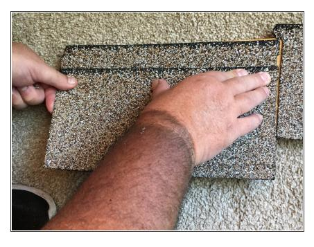
Slip the new shingle in place, and line it up where the old shingle previously was.
