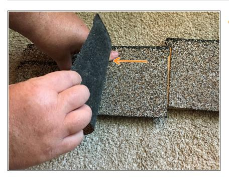
Remove the single broken shingle, carefully, without ripping out the shingles above.
