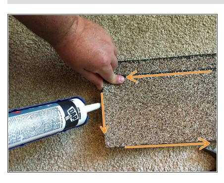
Slightly lift the edges of the shingle and apply a thin layer of cement along it.
