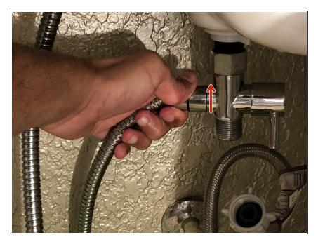
Unscrew the hose from the Tconnector by turning the knob counterclockwise.
