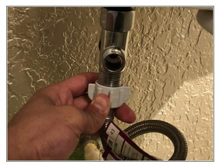
Screw the water supply nut onto the bottom of the T-connector by turning the knob clockwise. Make sure it is firmly hand tight.
