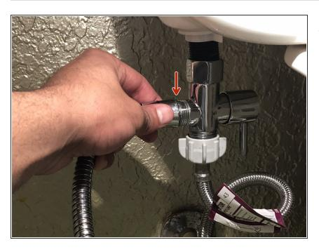
Screw the water supply hose back on the T-connector by turning the knob clockwise. Be sure not to over tighten the nut.
