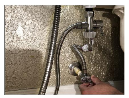
Turn off the toilet water valve by turning the knob clockwise.
