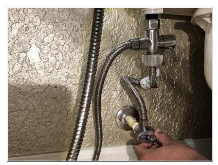
Turn on the toilet water valve by turning the knob counterclockwise. now, you can test your water and spray it through the hose. Make sure there is no water leaking.
