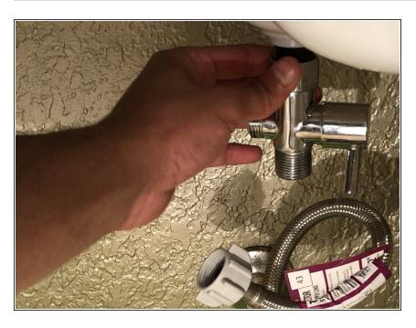
Unscrew the T-connector from the toilet by turning the knob counterclockwise.
