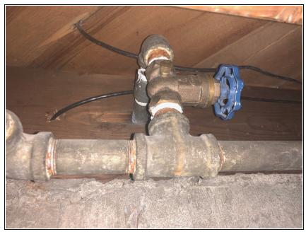
Find where the water supply feeds the sprinkler system and close the valve in the event of emergency or unforeseen circumstances.
