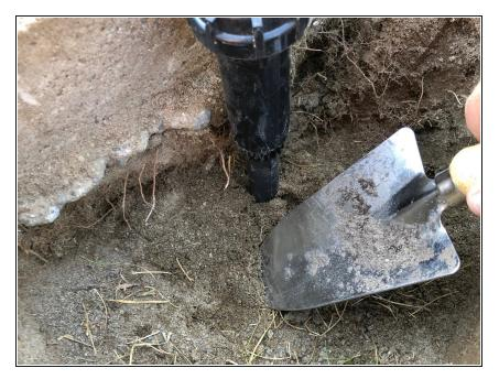
Using your hand or a gardening trowel, finish digging so that the sprinkler head is fully visible and is clear of dirt and debris.
