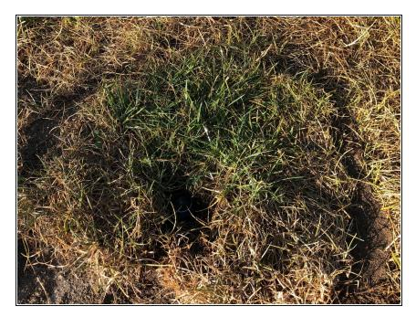
Fill the hole in and pack it down to avoid unwanted movement of the new sprinkler head.
