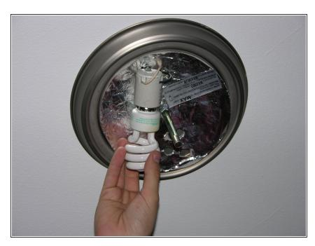
• Twist the light bulb out of it's socket.
