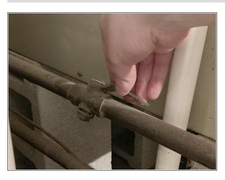
If you have a gas water heater, turn off the valve on the incoming gas line to shut off the flow of gas.
