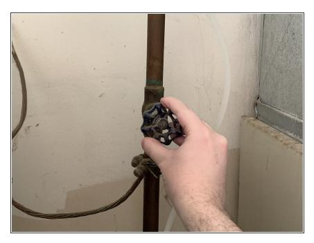
Shut off the cold water line going to the water heater.
