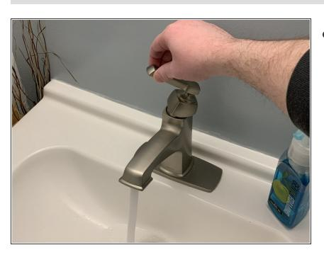
Turn on the hot water at a nearby faucet and leave it running to relieve any pressure in the tank and vent the water heater as it drains.
