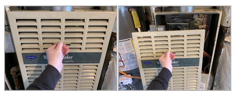
Grab the handle on the front panel marked "Lift" and push up to release the panel. Place it off to the side.
