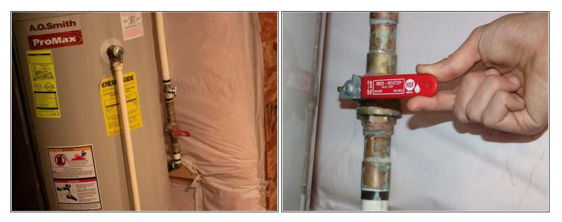
• Shut the water supply off to the irrigation system. (usually found in the utility room or basement)
