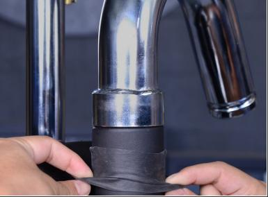
Peel the rubber sleeve down from the elbow pipe to reveal the pipe socket.
