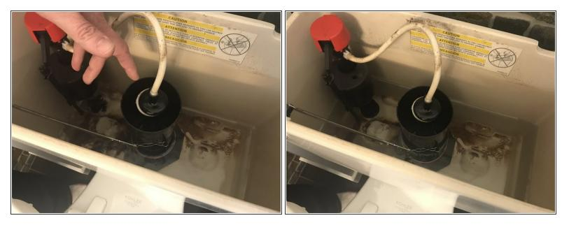
Release the float and the valve seat, and allow them to fall back into place. The flow of water will resume.
