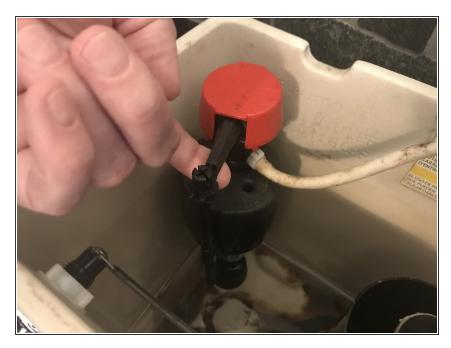
Gently lift the float up, ending the flow of water. This will prevent the toilet tank from refilling.
