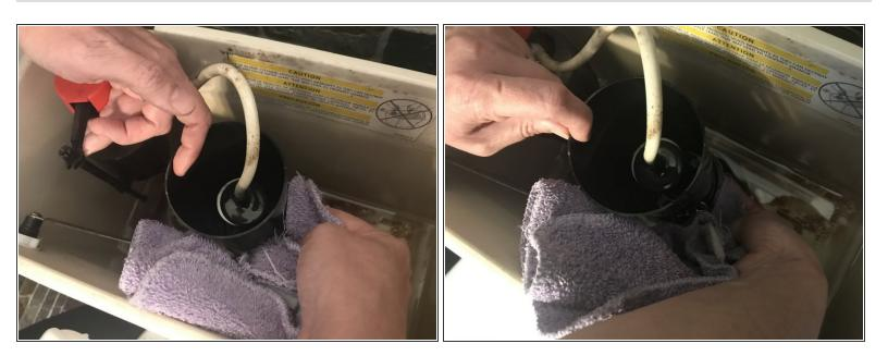
Wipe the valve seat with a rag or towel to remove the calcium deposits. Don't forget to wipe the bottom of the valve seat, as deposits can form there as well.
