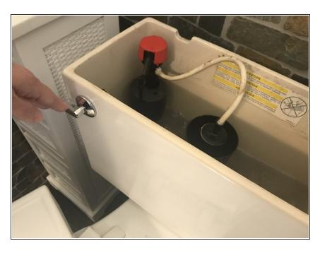
Flush the toilet, and hold down the flush lever until the tank is completely empty.
