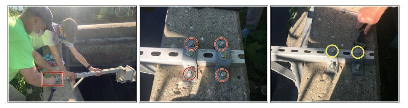
• Using an adjustable or socket wrench, remove the four 3/4" nuts and washers from the U-brackets attaching the long strut channel to the bridge.
