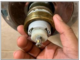
• Use your hands to turn the ring to the left to loosen it. If the ring is not turning then use a wrench.
