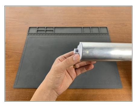
• Replace the bearing cap and nub on the left side of the shade tube.
