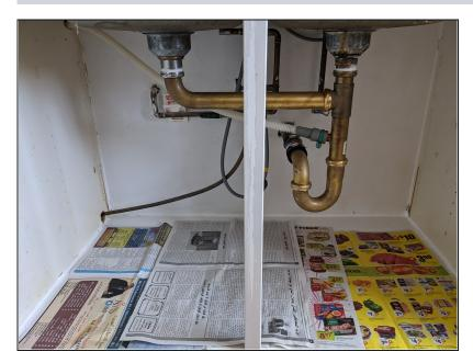
Clear out the area for easy access. Place a disposable mat under the sink to make cleaning easier.
