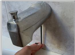
Retighten the set screw using the 5/32" Allen key.
