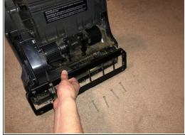
Using your Phillips #2 screwdriver, remove all four 42 mm long screws from the bottom plate of the vacuum.
