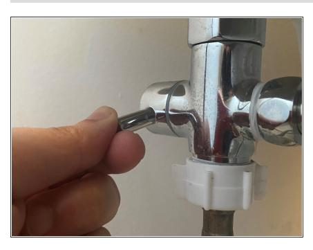
Push this valve downwards to shut off the bidet sprayer.
