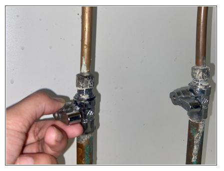
Turn the water shutoff valve underneath the sink downwards to stop the flow of water.
