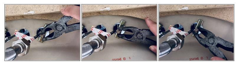
• With pliers, tighten the mounting nuts underneath the sink in the same location they were removed from.
