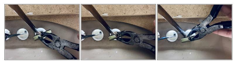
• With pliers, unscrew the mounting nuts underneath the sink by turning them counterclockwise.
