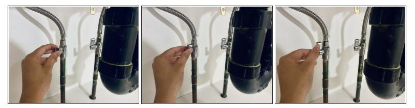
• Turn the shutoff valve upwards to line it up with the pipe and resume the flow of water.
