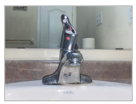
• Turn the tap(s) on to release any pressure build-up in the pipes.
