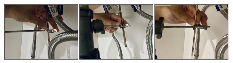
• Reattach the lift rod for the drain plug by lining up the holes and pushing it through the metal rod.
