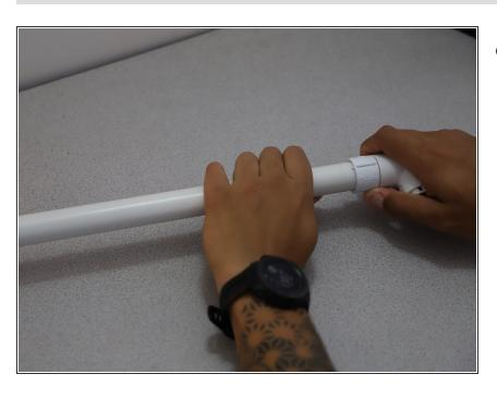
Hold the pipe in place firmly for a couple minutes until it is completely sealed and dry.
