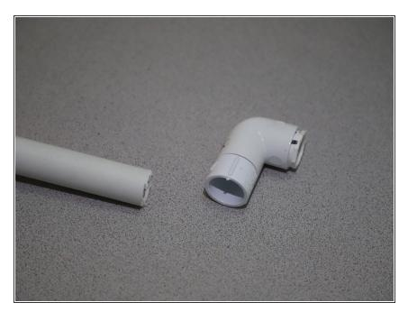
Make sure the adapter fits the broken end of the water pipe by fitting the adapter without the sealing glue. (Just in case it is not the correct measurement.)
