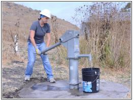
Perform a water test on the pump, by raising and lowering the handle a full 40 strokes. A properly performing pump will yield greater than 10 liters.
