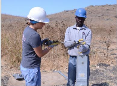
While holding the pump rod below the first connection tightly, lower the first portion of the rod to a horizontal position.
