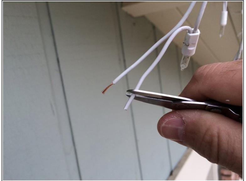
**⚠** Make sure the lights are completely unplugged from any electrical sockets before proceeding further.
