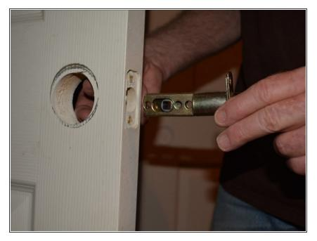
• Remove the latch face plate and latch mechanism.
