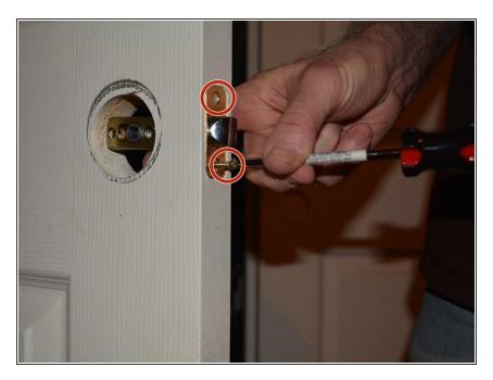
Unscrew the two short screws on the latch face plate.
