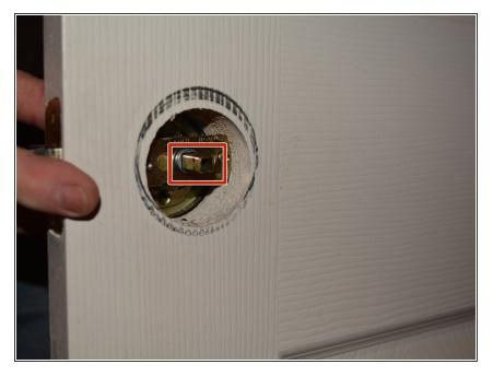
You will see the latch face plate (the rectangular piece of metal) where the latch of the door knob is located.
