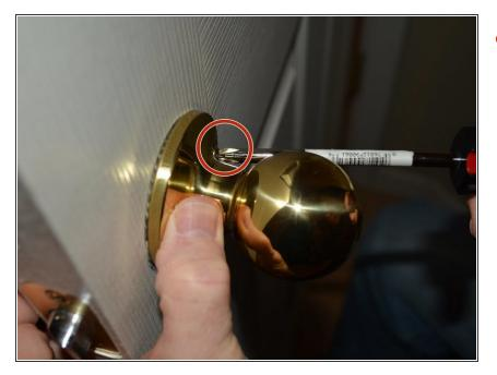
Screw in both long screws on both sides of the door knob.
