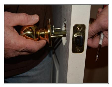
• Remove the door knob on both sides of the door.
