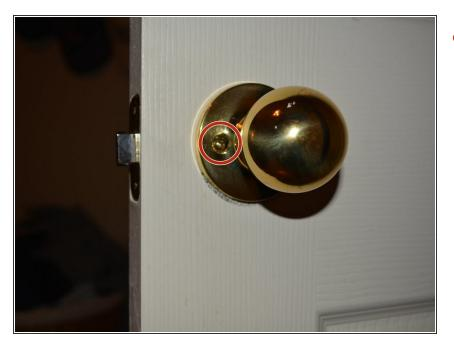
Face the inside of the knob, you should see two Phillips head screws on either side of the central knob.
