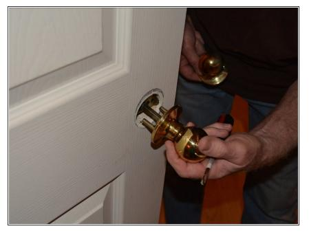
Insert the door knob that goes on the inside of the room, aligning the peg and screw holes with the threaded cylinders of the latch mechanism.
