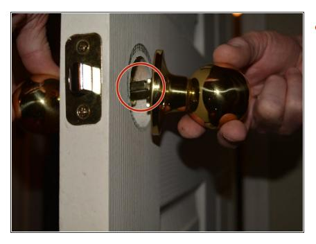
Align the door knob that goes on the outside of the room, aligning the peg and screw holes with the threaded cylinders of the latch mechanism.
