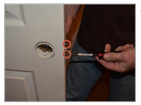
Screw in both short screws of the latch face plate.
