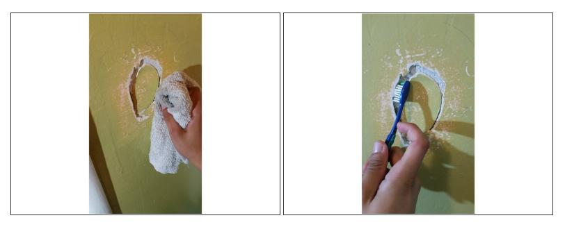
• Use the rag and the toothbrush to clean off any excess rubble near the hole.
