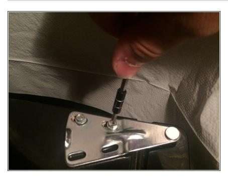
Use a JIS #1 screw driver to remove both 25mm bolts that are attaching the door to the refrigerator.
