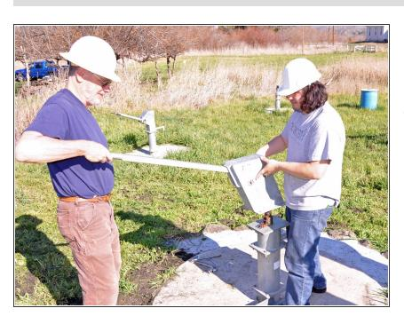
Lift the pump head off of the water tank and place in a sanitary place, preferably above ground, to prevent contamination.
