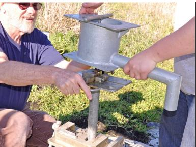
Turn the water tank counterclockwise until it comes free from the pipe.
