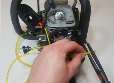
Cut both of the fuel lines flush (removing the angle that was previously cut).
